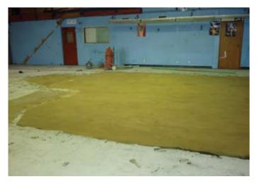
The challenge for Topcoat was to transform a pitted and delaminated concrete base into a glossy new floor of showroom standard.
